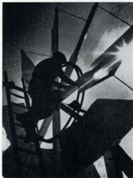
Repairs being carried out to the fantail
